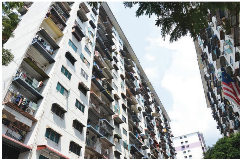
The repainted flats look cheerful and bright with a new coat of paint.
